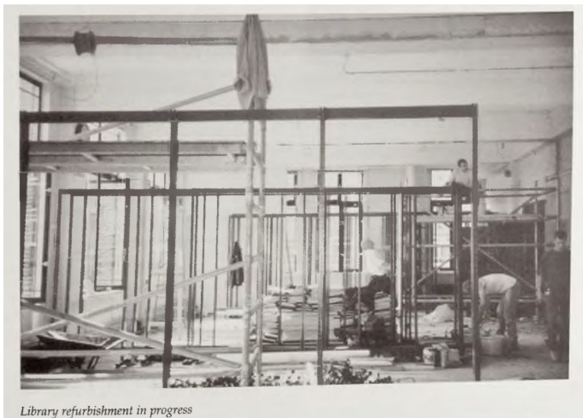
Library refurbishment [UCL ION Annual Report 1994-1995, p.135. QSA/19005]
